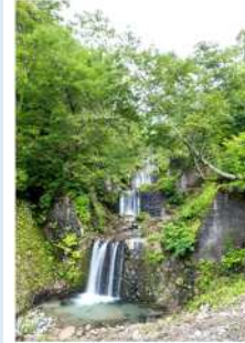
Dorodani Sabo dams (Built 1930 - 1938)
