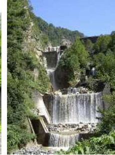
Shiraiwa Sabo dam (Built 1929 - 1939)
