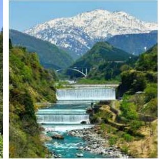
Hongu Sabo dam (Built 1935 -1936)
