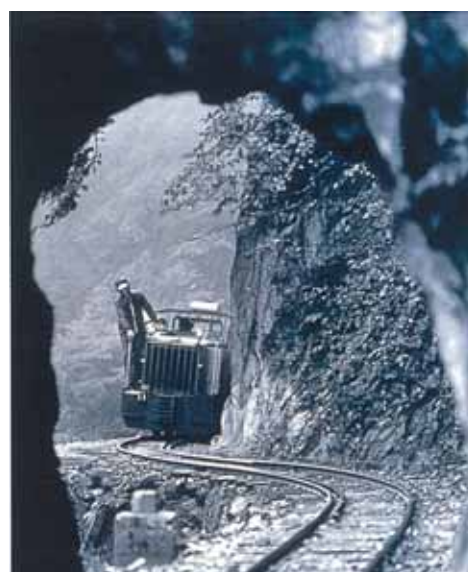
One of the trollies which have ferried people and materials during the 80 years since construction started in 1927
