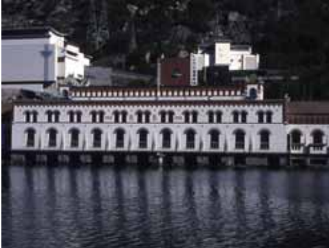
Hydro power station (Norway)
