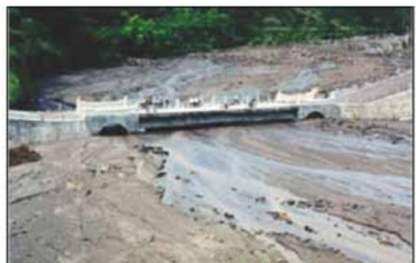
b). After debris flow occurrence
